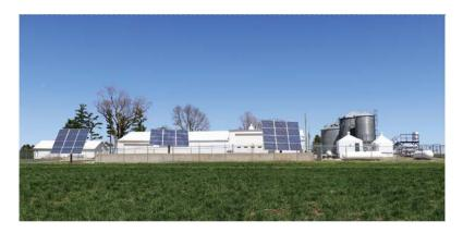
**CARBON-FREE FARMING:** Creating fuel and fertilizer on the farm requires a lot of interconnected parts. Behind the solar panels, a long, squat building houses the tractor and control equipment; two small white huts house the ammonia generator and hydrogen pumps. The white tanks in front of them store the generated nitrogen and hydrogen, while the large gray tanks store additional hydrogen at high pressure. To the far right are the steps and railings of the tractor fueling dock.
