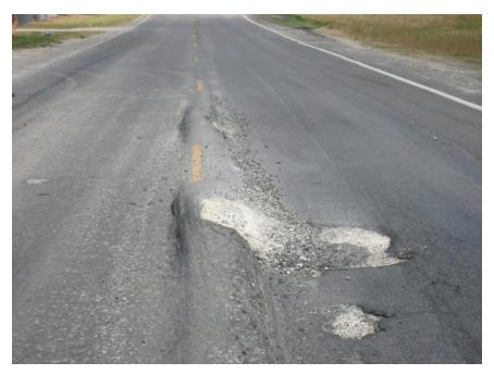
**FIGURE 7-3** Pavement shoving, loss of surface (IH 35W – frontage road) SOURCE: Quiroga et al., 2012.
